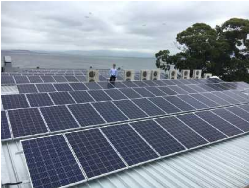
Figure 9: Stage 1 installation of solar panels at Illawarra Yacht Club
